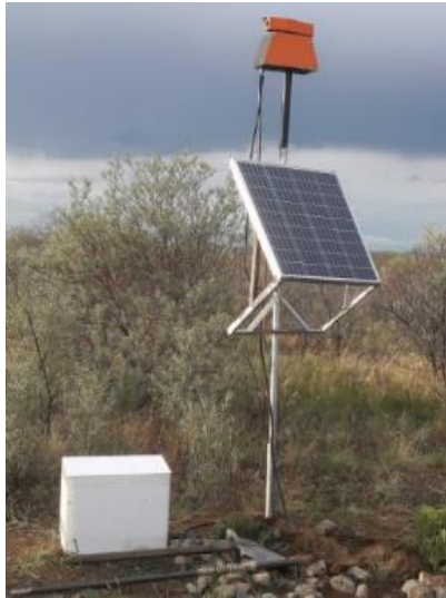
Figure 3. Existing bird repellent equipment in the field
